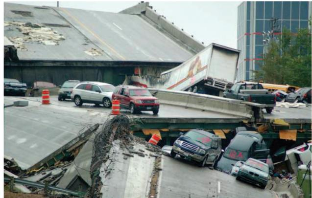
Fig. 9 - I35W, crollo del ponte sul fiume Missisipi, Missouri (2007). *I35W, collapse of the bridge on the Missisipi river, Missouri (2007).*
