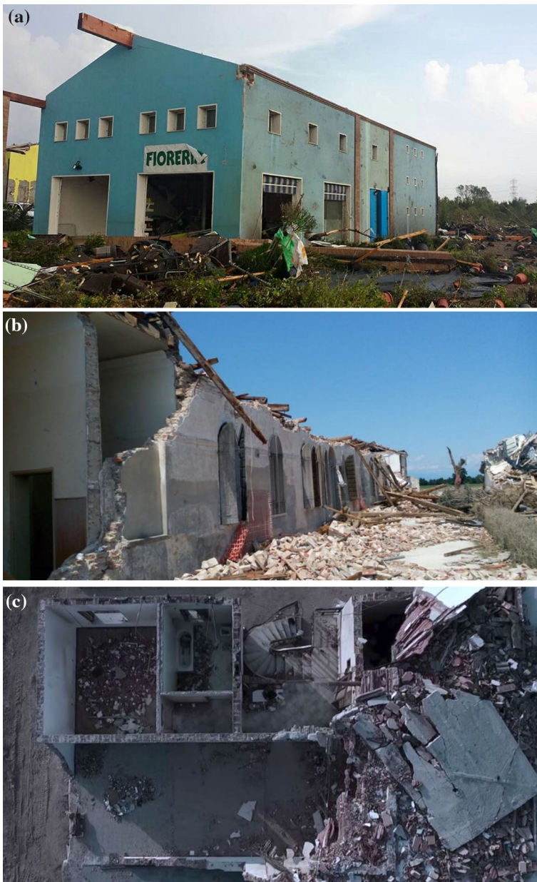
Fig. 20 Incremental damage observed in the recent Italian events: a translation or sliding; b overturning; c racking; d material/component failure; e incoming collapse; f total destruction
